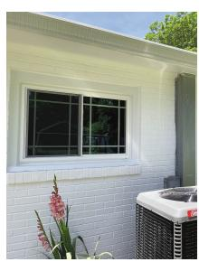
Sliders come in 2- and 3-lite models. 3-Lite Sliders have a center fixed panel and are available in configurations of 1/3-1/3-1/3 and 1/4-1/2-1/4.
